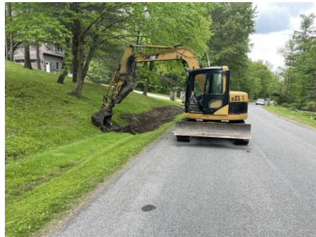
Performing Drainage Swale Maintenance on East Hyerdale Dr.
